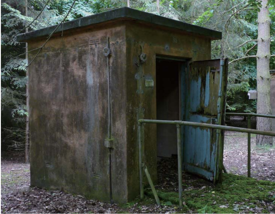
FIGURE 10 Igloos at RAF Banham Special Storage Unit were used to store the plutonium cores. This is number 35. The large number of igloos may have been designed to intimidate and impress as it is unlikely they were all used either here or at Faldingworth.
